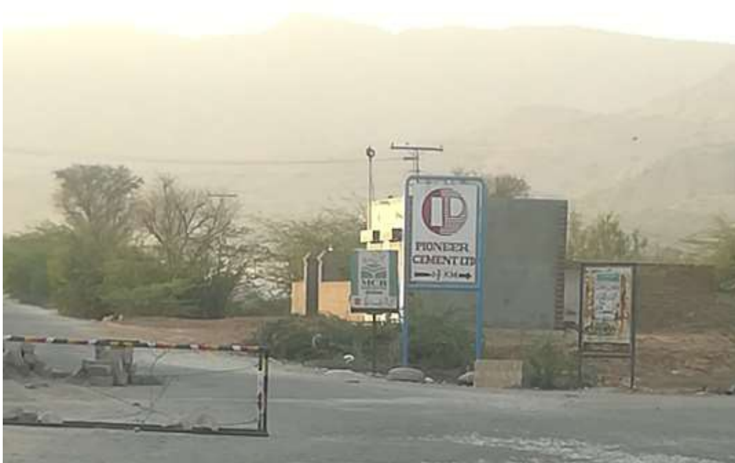
A cement factory
